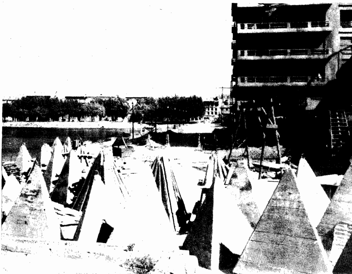
Figure 19.—Concrete tetrahedra used as antitank obstacles.
