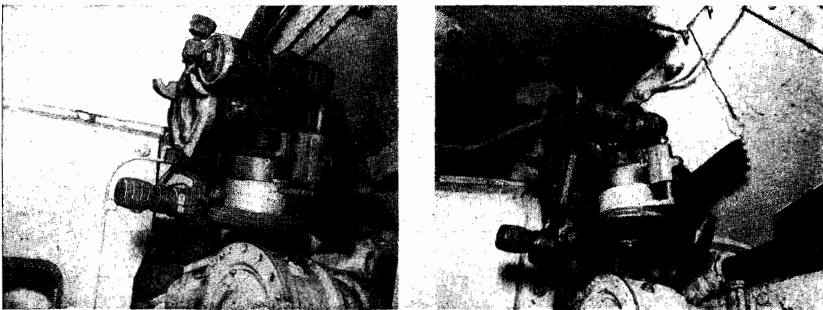
Figure 14.—Sight mounts (Left) For 7.5 cm (Stu. K40) Pz. Kpfw. III chassis. (Right) For 7.5 cm on Pz. Kpfw. III w/o rotary cupola.
