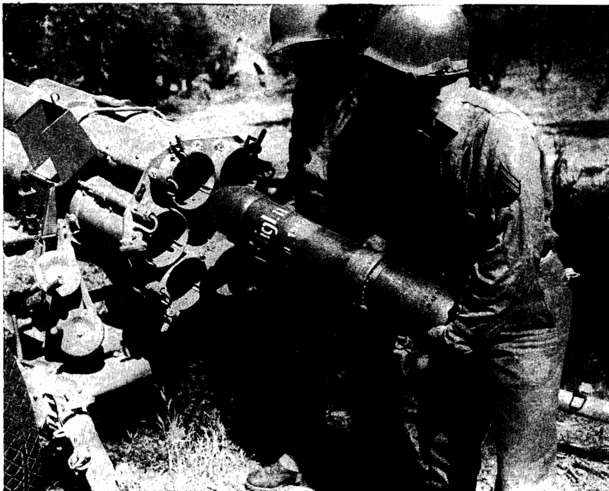
Figure 127.—15 cm Nebelwerfer 41 being loaded.
