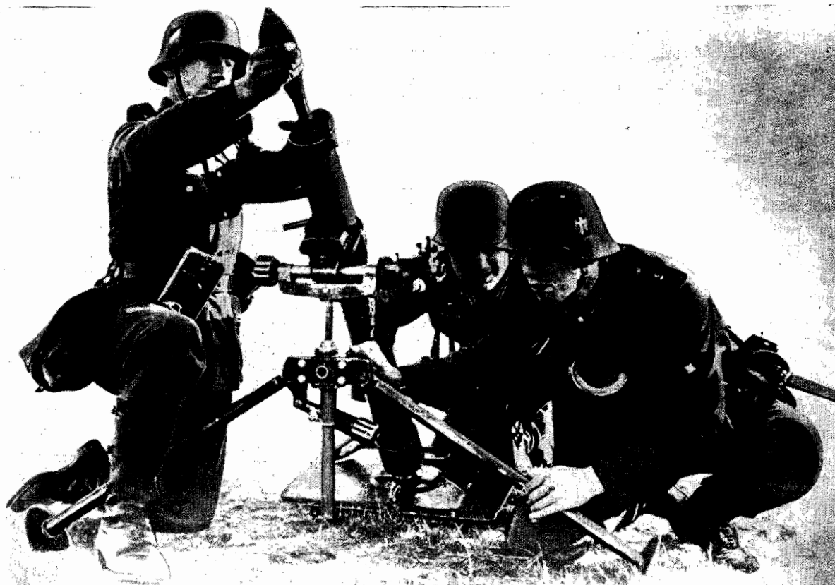
Figure 23.—8 cm schwerer Granatenwerfer (81-mm mortar) in action.
