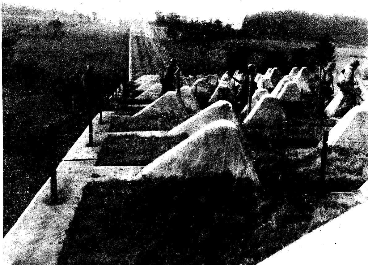
Figure 16.--Dragon's teeth showing concrete foundations.
