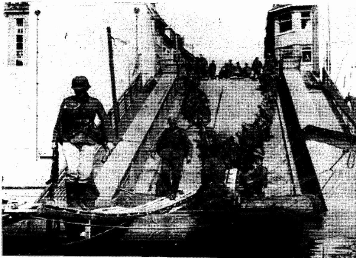
Figure 96.—Track bridge and medium pneumatic boat.
